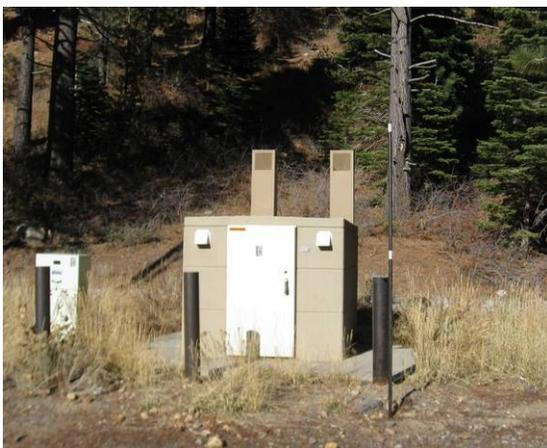
Figure 11, Controlled Environment Cabinet
