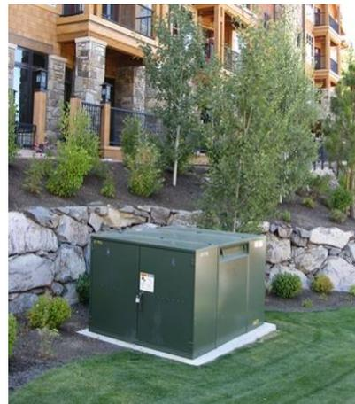
**Figure 5, Pad Mounted Switch**
