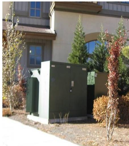
**Figure 4, Three Phase Transformer**
